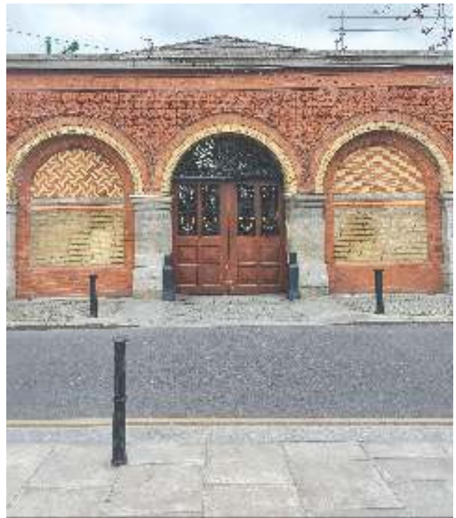
2. The Dublin Fruit Market, north facing façade featuring brick and tile.
